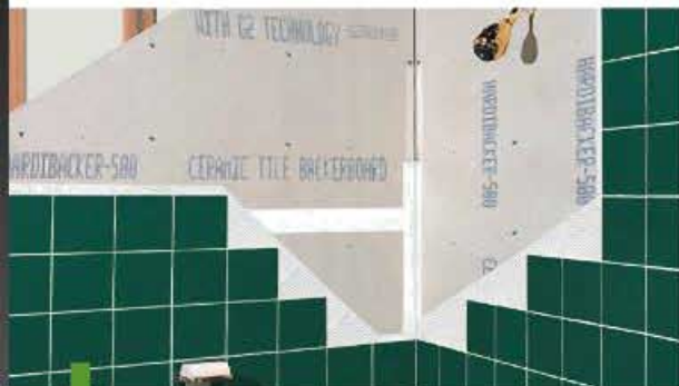
HardieBacker installed in a shower. Photo courtesy of James Hardie.
