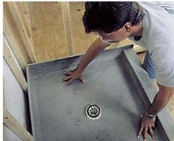
I've never been fond of using rubber liner systems for creating a tiled shower pan. Most of these systems are built incorrectly and that can result in leaks and mould build-up. [Redi Pan](#) builds a prefabricated shower pan that is rigid, one piece and pre-sloped. What makes this pan different is that you can tile directly onto it. This allows you to create that custom tiled look with a perfect consistent slope that is leak proof and mould free.
